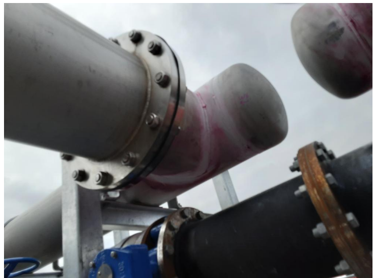
Image 4 of 7 - Spool #2 weld 4-6
