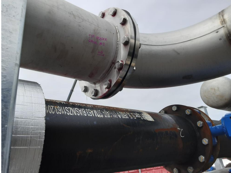
Image 1 of 7 - Spool #3 welds 8
