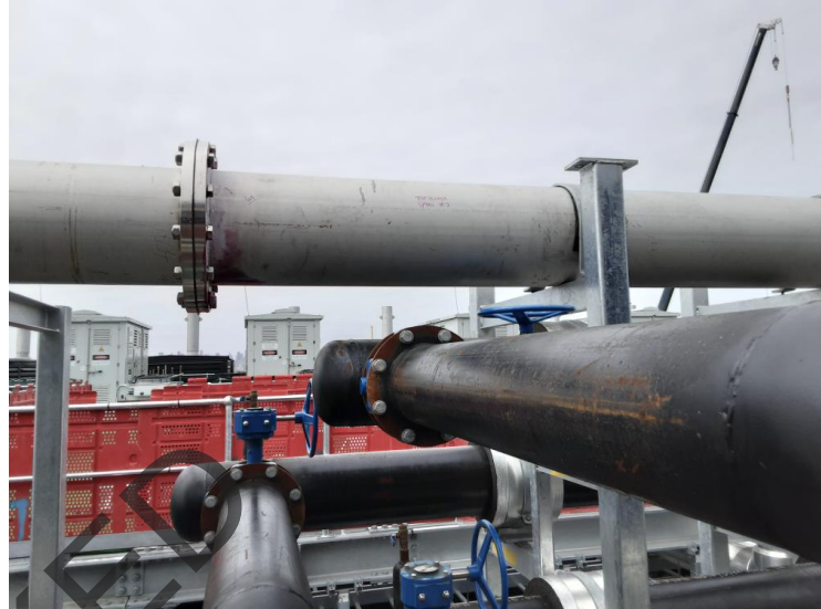
Image 6 of 7 - Spool #2 weld 1
