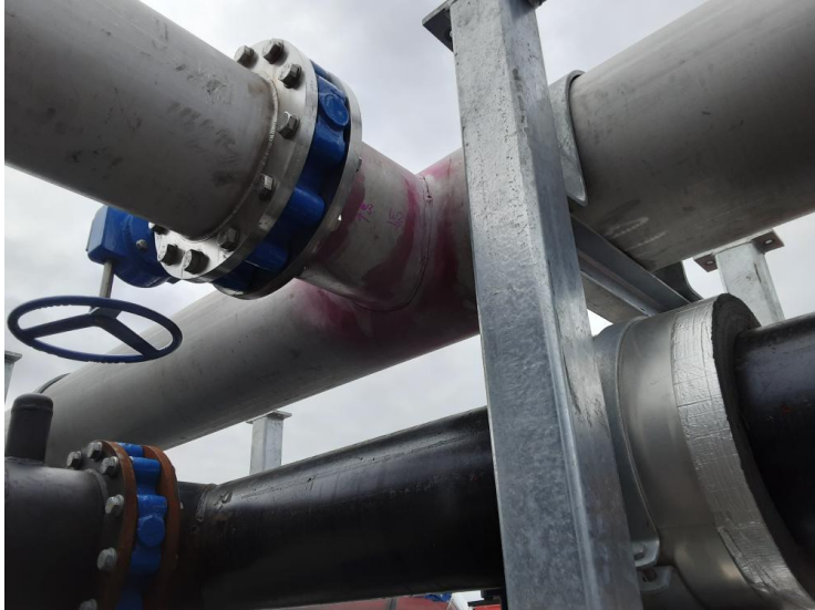
Image 5 of 7 - Spool #2 weld 2 & 3
