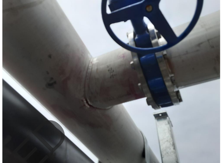
Image 2 of 7 - Spool #3 welds 6 & 7
