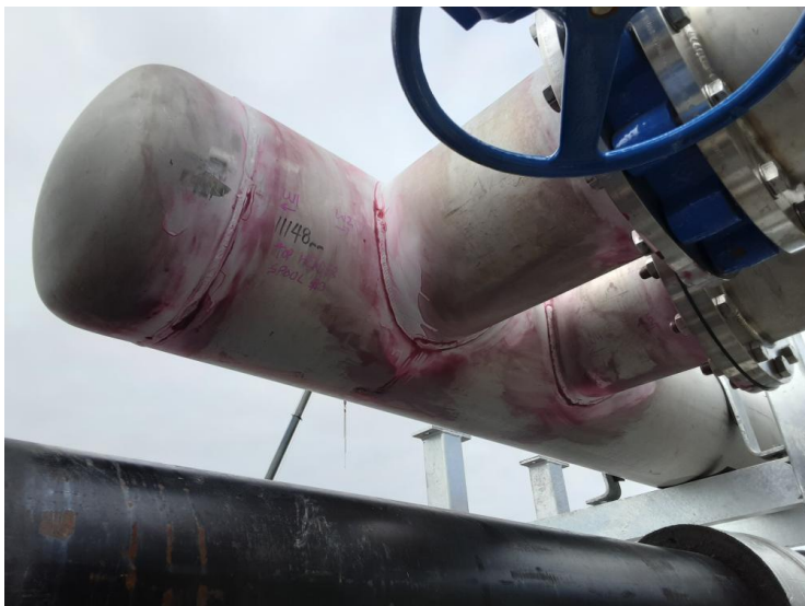
Image 3 of 7 - Spool #3 welds 1-5
