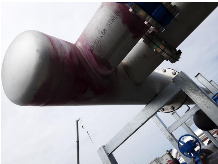
Image 7 of 7 - Spool #1 welds 1-5
