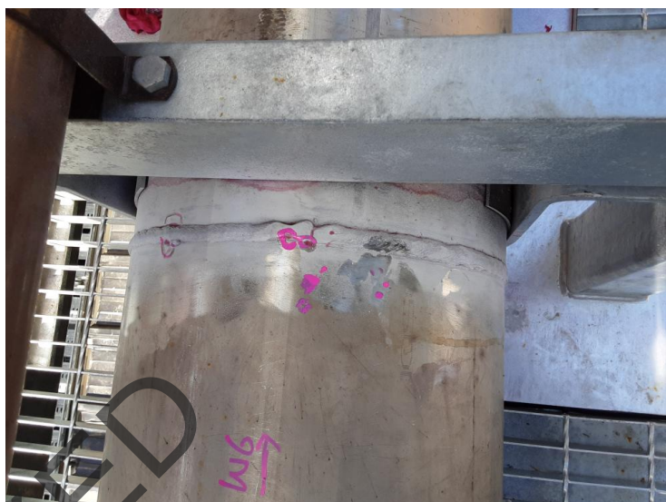
Image 6 of 12 - South end spool #2 W6
