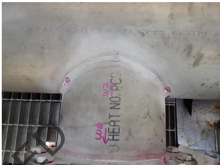
Image 10 of 12 - South end spool #1 W7-8
