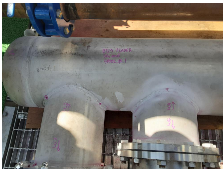
Image 12 of 12 - South end spool #1 W1-5
