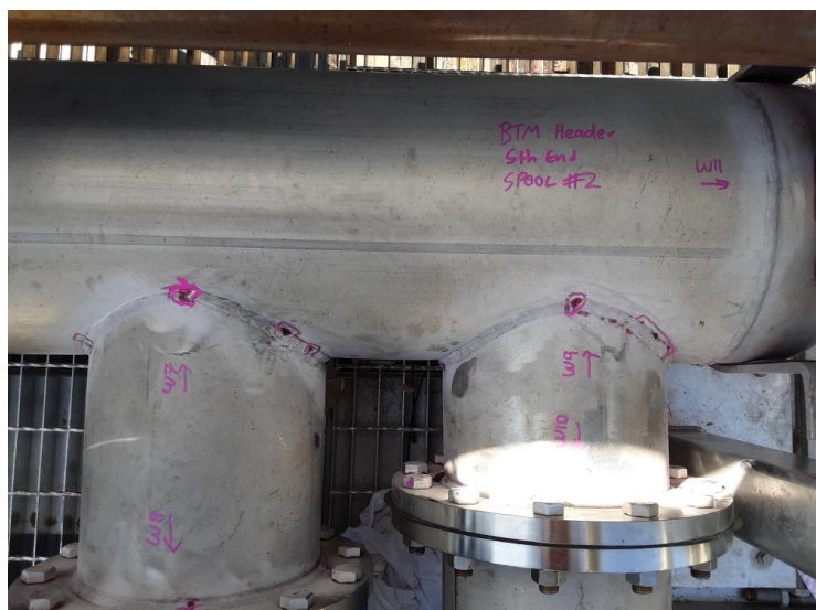
Image 5 of 12 - South end spool #2 W7-11
