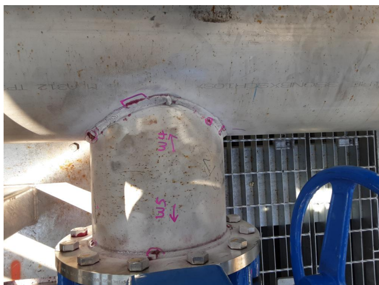
Image 7 of 12 - South end spool #2 W4-5
