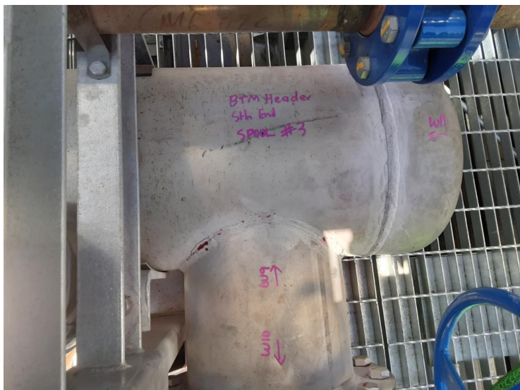
Image 1 of 12 - South end spool #3 W9-11
