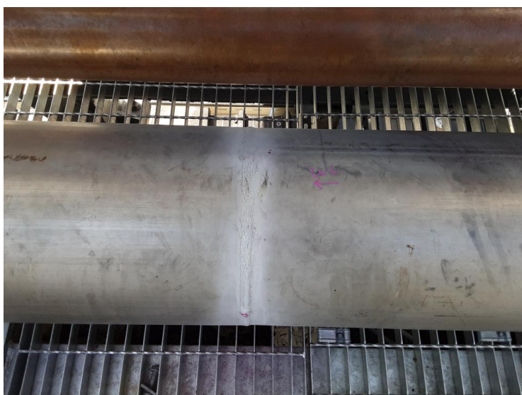
Image 11 of 12 - South end spool #1 W6
