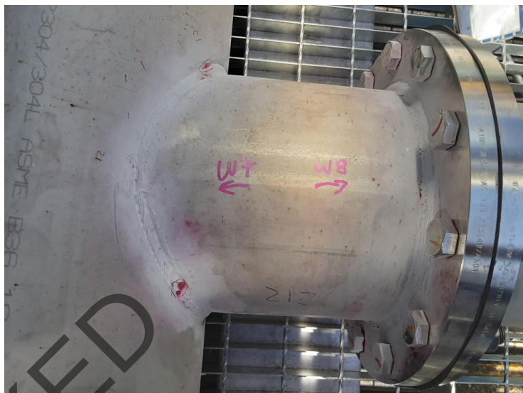
Image 2 of 12 - South end spool #3 W7-8
