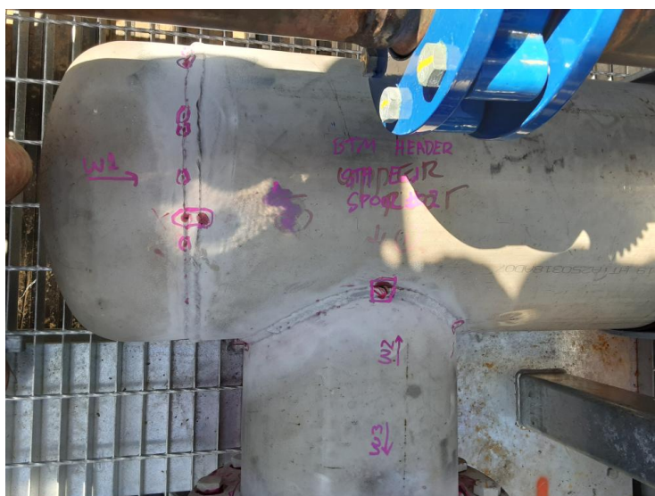
Image 8 of 12 - South end spool #2 W1-3
