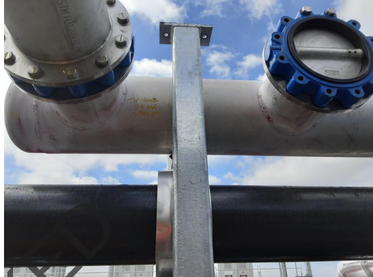
Image 6 of 6 - Top header South end spool #4 W1-5
