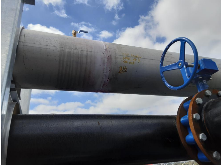
Image 5 of 6 - Top header South end spool #4 W6
